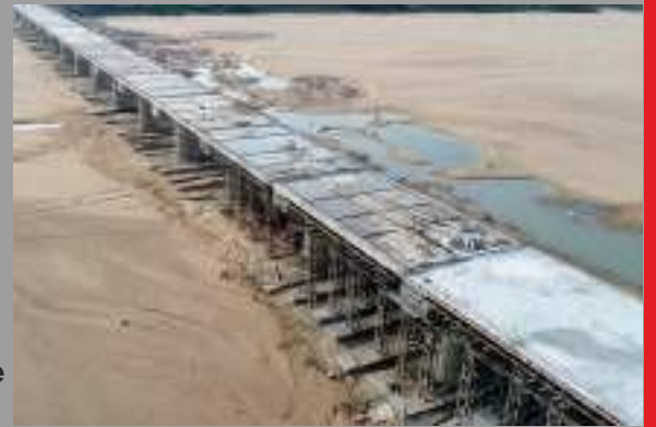
Khaira Bridge , MP
