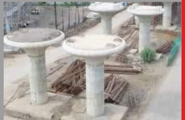
Railway Overbridge Rewa, MP
